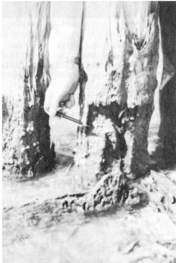
Base of piling showing gross destruction to wood caused by gribbles, Limnoria .
