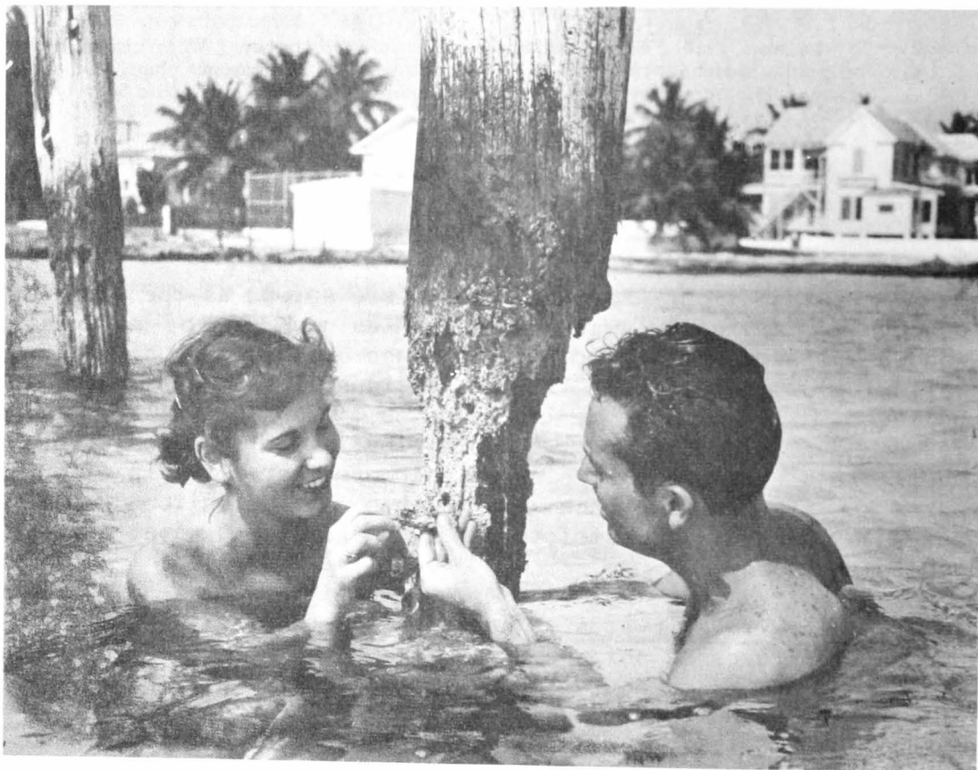
Piling ravaged by gribbles. Unlike the shipworm, this easily spotted marine borer attacks the surface of wood, destroying it layer by layer. Photograph by Robert F. Sisson, credit: National Geographic Society.
